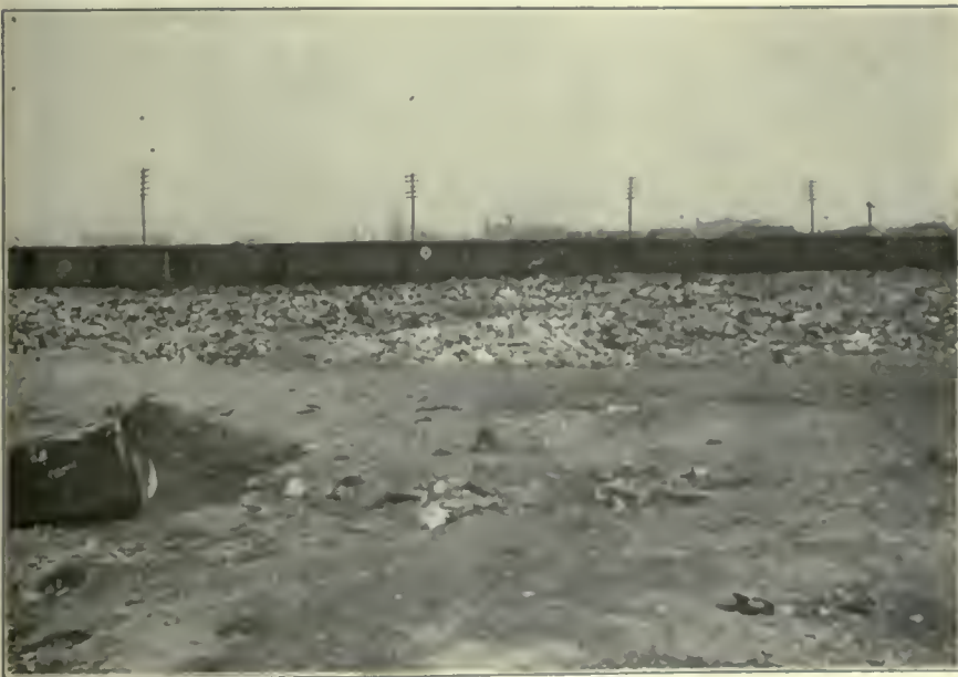
FIG. 56. REFUSE DUMPS, A SOURCE OF DUST. Street sweepings are frequently used for filling in low ground. This view illustrates such a case and shows conditions favorable to the development of dust. The dump here shown is located within a block of one of Chicago's boulevards.
